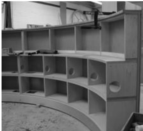
Reception desk being fabricated
